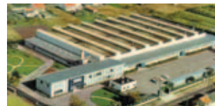
Nantes, France R&D and Marketing excellence centre. Application centre for customised solutions and assembly of CP electric tools and assembly systems.
