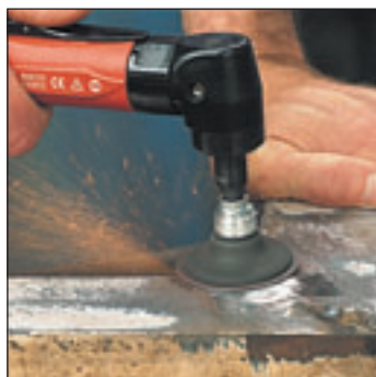
PLANING DOWN WELD
